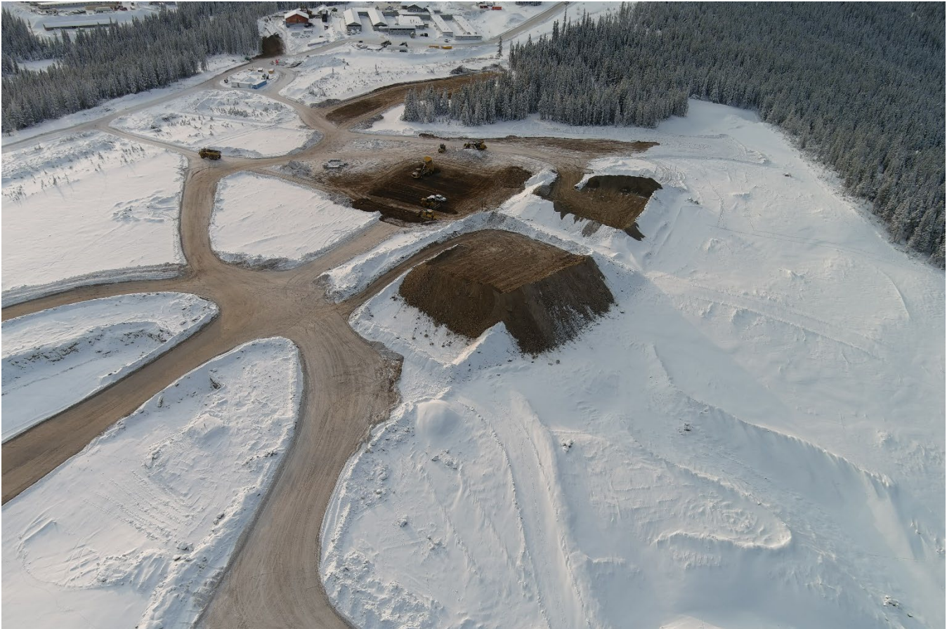
Figure 1: Blackwater Project Plant Site Area (Looking South/West) Q4-2022
