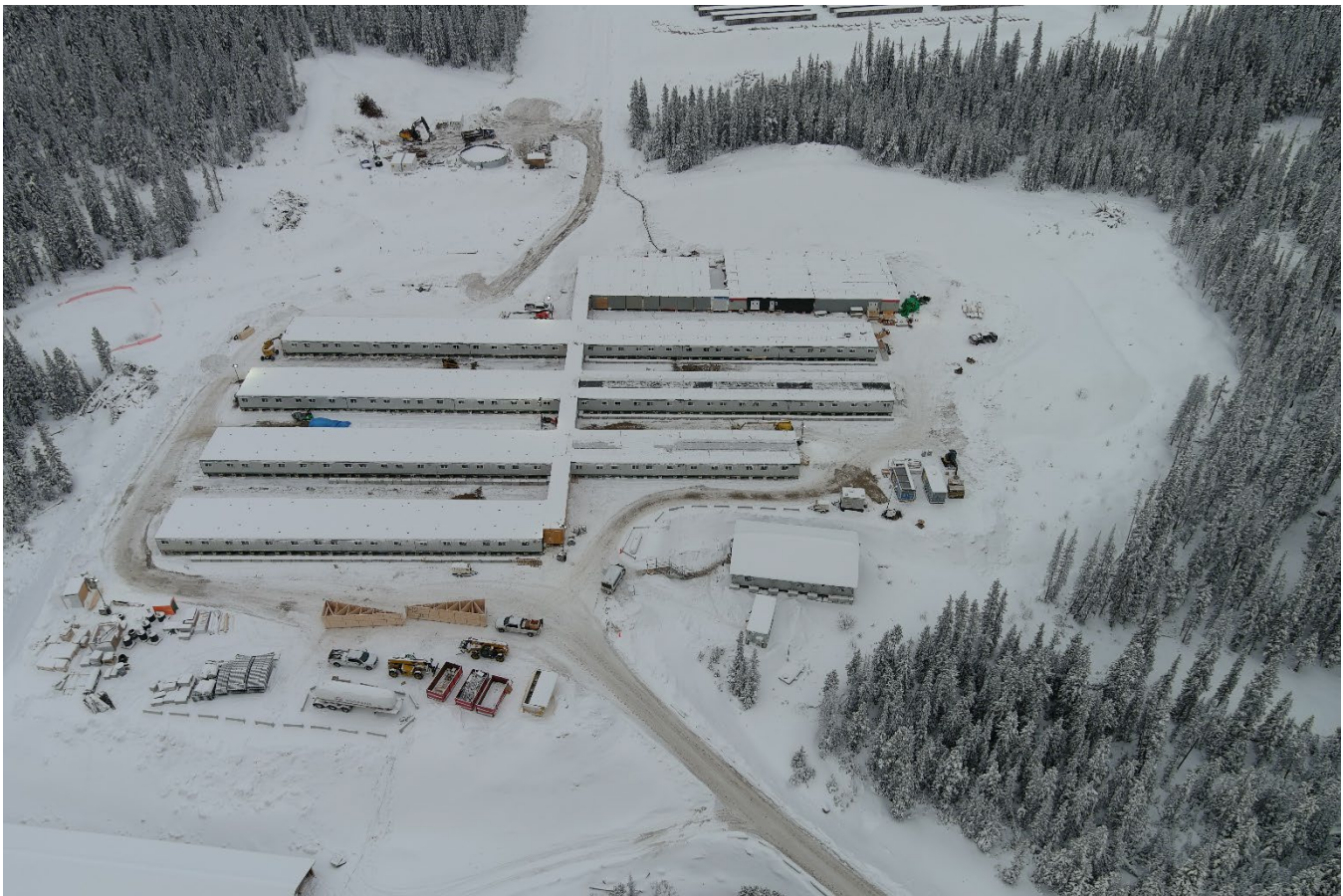
Figure 2: Blackwater Project New Construction Camp Area (Looking South) – Q4-2022
