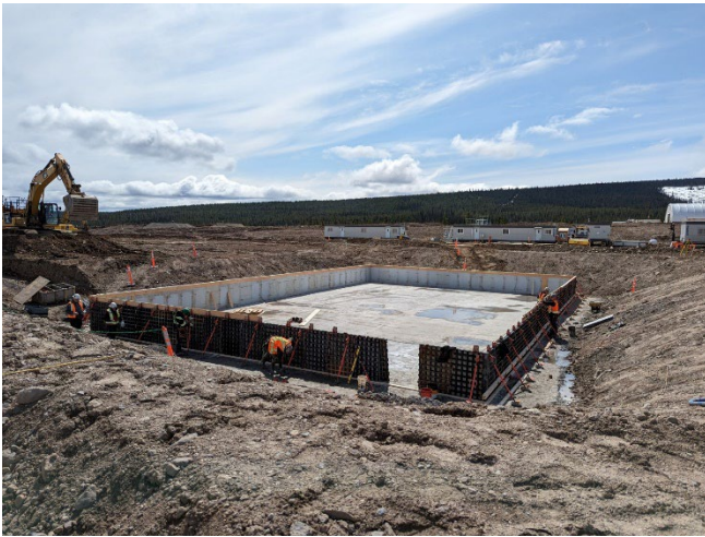
Ball Mill Foundation Formwork Installation- May 2023
