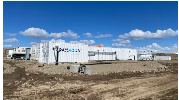
Wastewater Treatment Plant - April 2023
