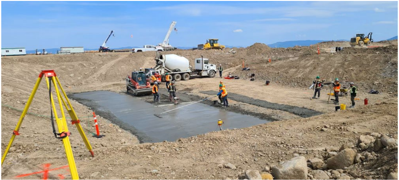
Ball Mill Foundation Blinding – May 2023
