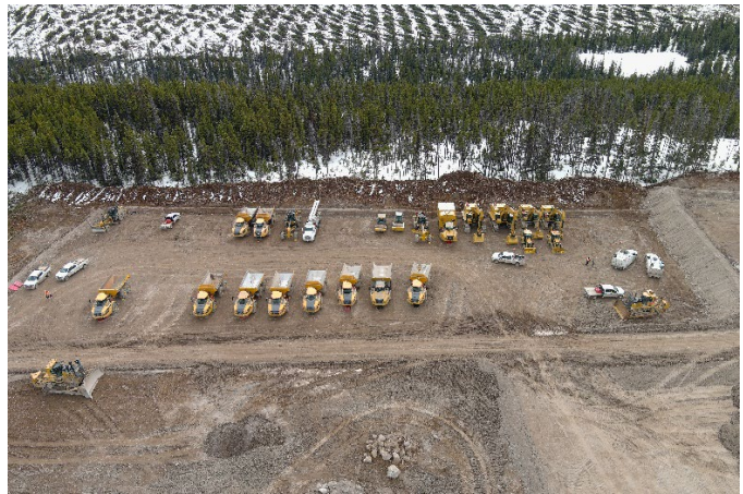
Construction Fleet at Blackwater Mine - April 2023
