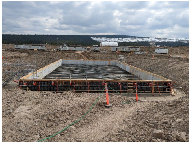
Ball Mill Foundation with rebar - May 2023
