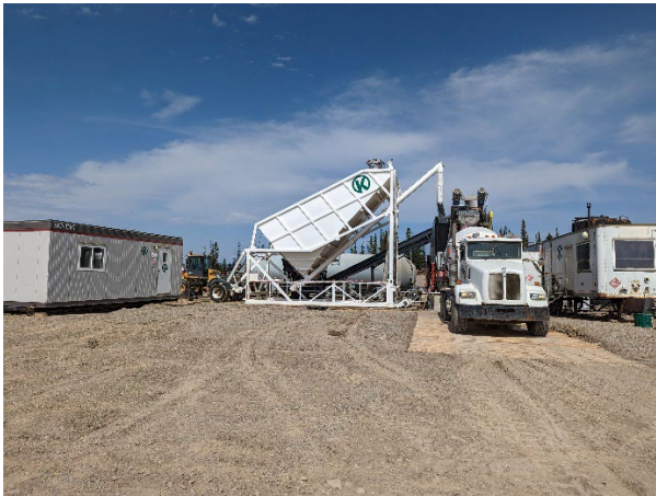
Concrete Batch Plant - April 2023
