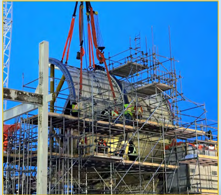
Ball mill shell installation - January 2024
