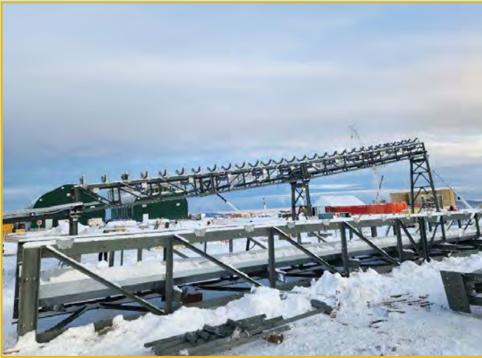
Conveyor assembly - January 2024
