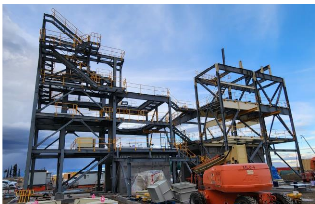
Secondary and tertiary crusher structural steel – October
