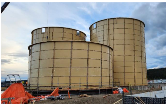
CIL tank construction – October
