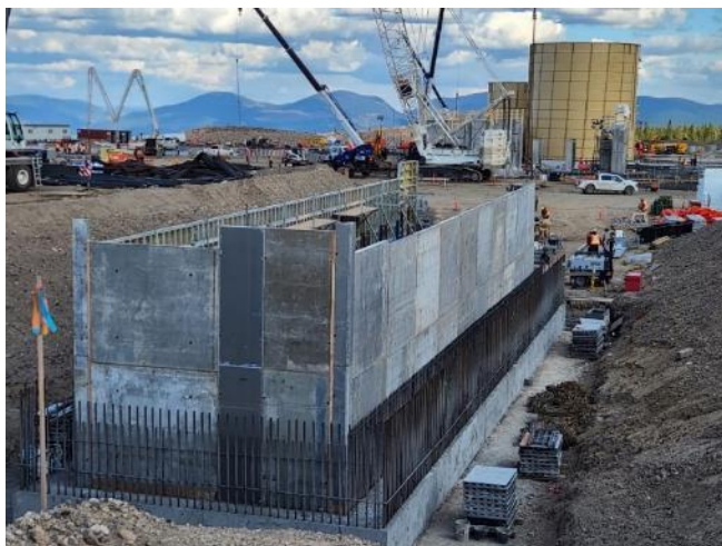
Reclaim tunnel – civil works – September
