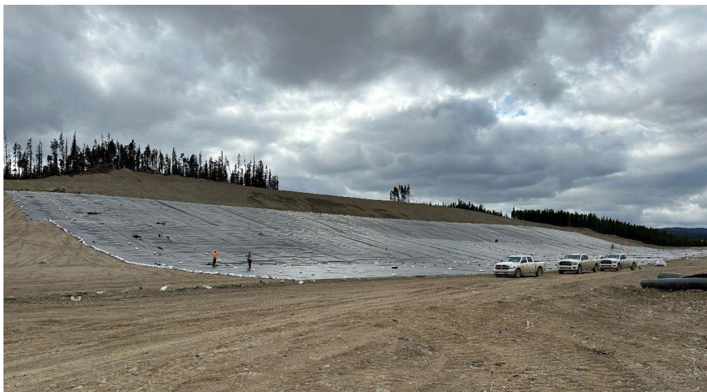
Water management pond creek diversion HDPE liner progress – September
