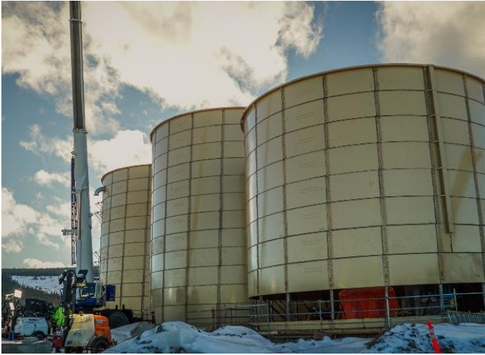
Tank Construction – December 2023
