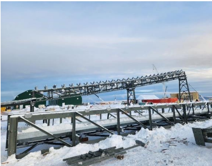
Conveyor Assembly – January 2024
