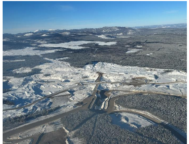
TSF Earthworks – January 2024
