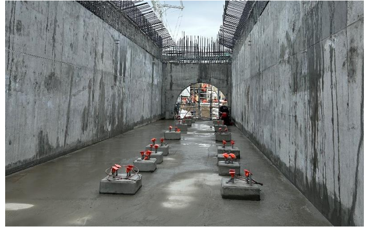
Interior Reclaim Tunnel – January 2024
