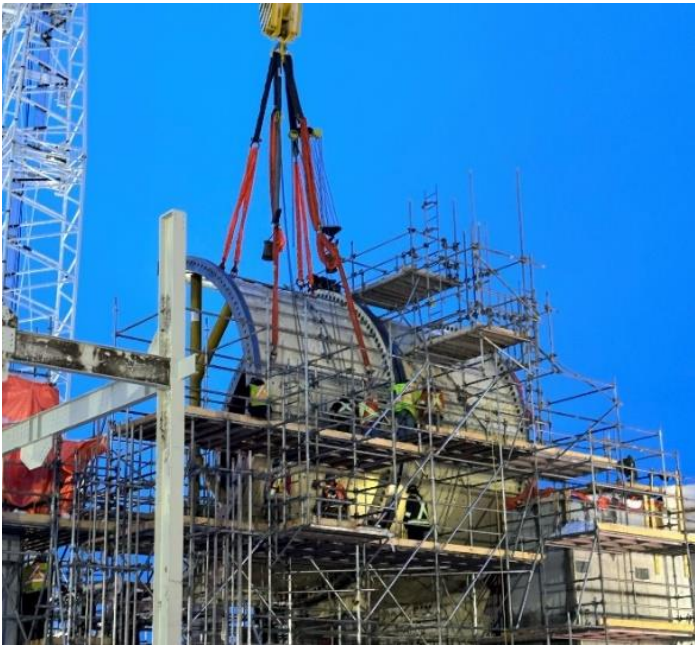
Ball Mill Shell Installation – January 2024
