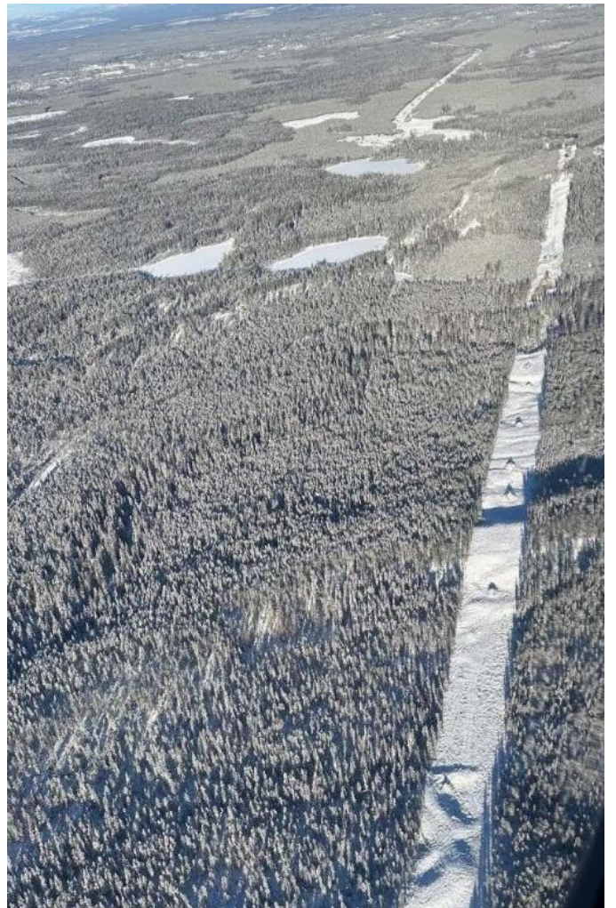
Transmission Line Clearing – December 2023
