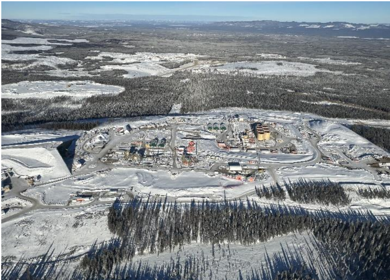
Project Plant Site – January 2024
