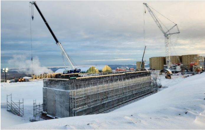
Exterior Reclaim Tunnel – January 2024
