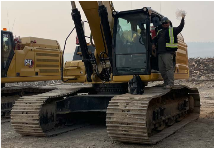
Henry Lopez, from Quesnel, removes the plastic seat cover and is the first operator of this excavator
