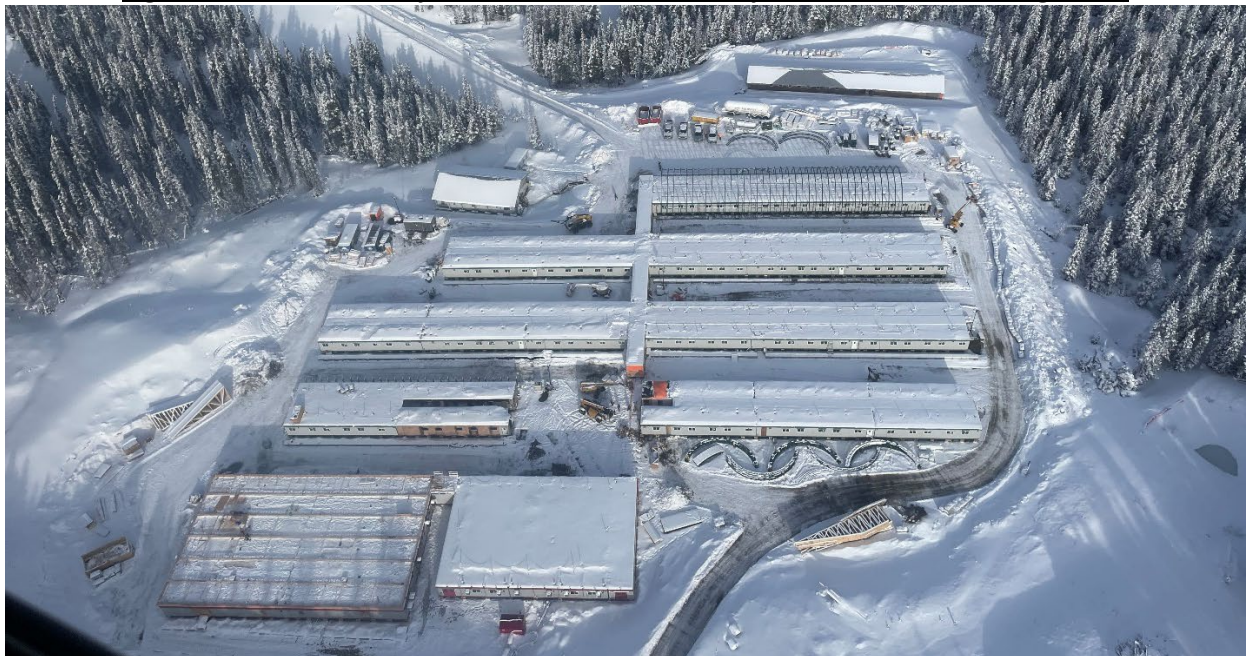
Figure 2: Blackwater Project New Construction Camp Area Q1-2023 (Looking West)
