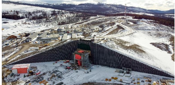
Primary Crusher Vault and MSE Wall
