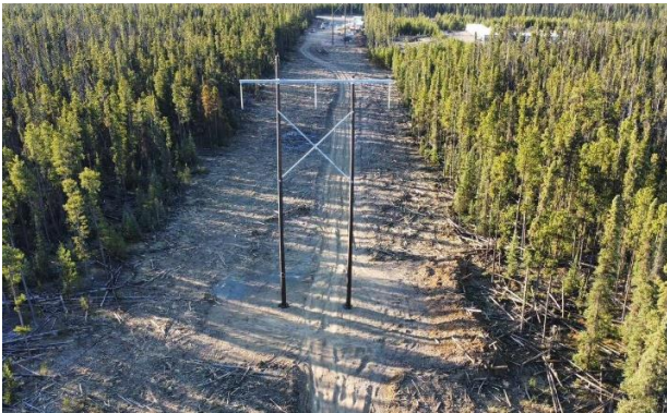
Transmission Line Construction
