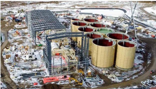
CIL Tanks and Processing and Reagents Buildings Installation
