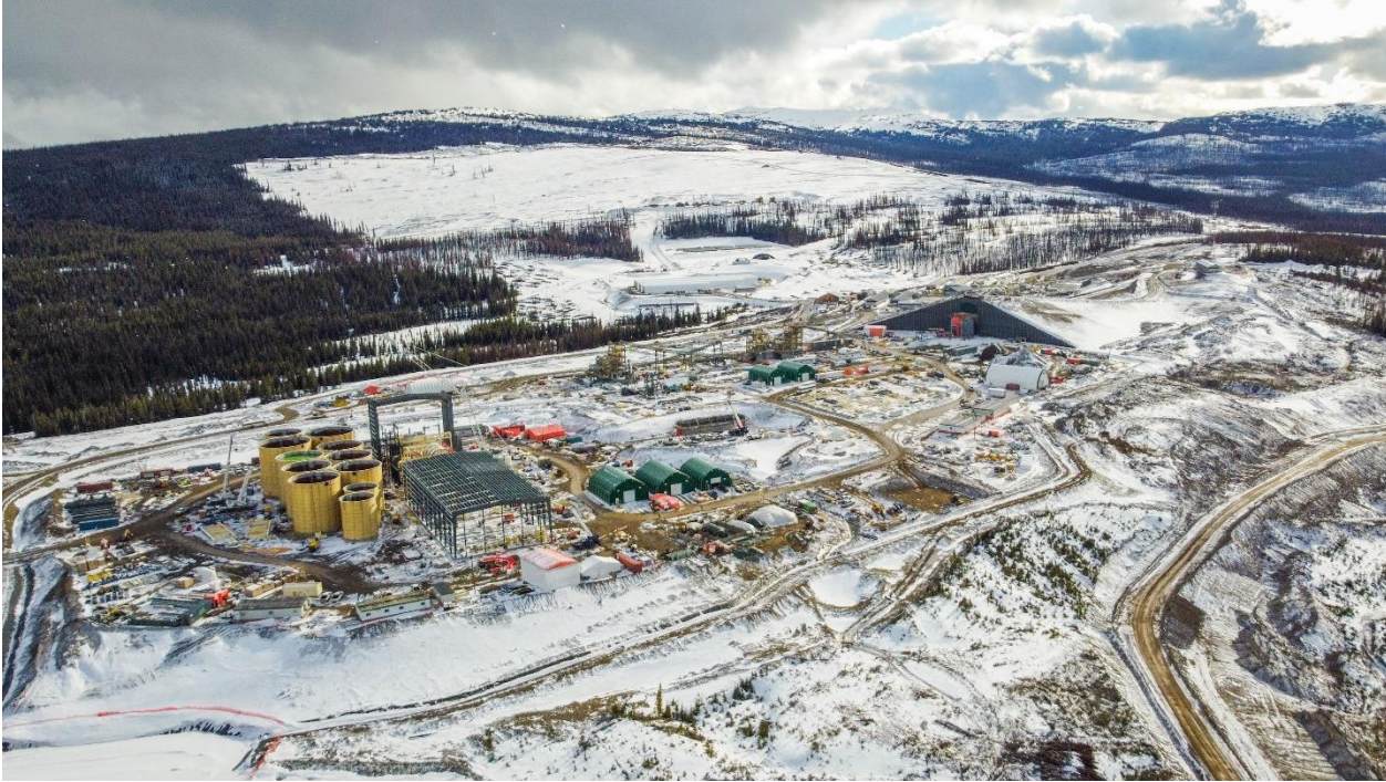
Project Plant Site – April 2024
