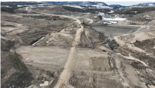
Earthworks at the Tailings Storage Facility
