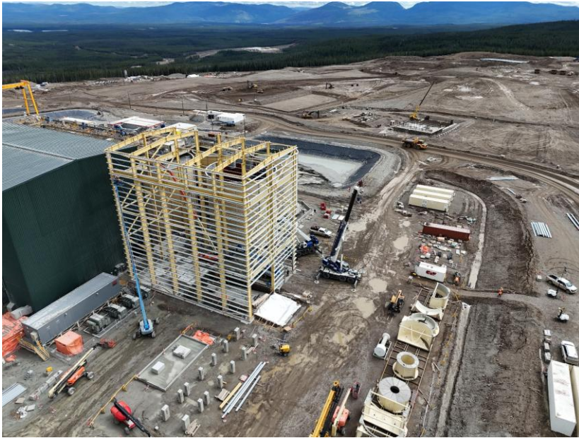
Figure 1 - Vertimill building construction – July 2026
