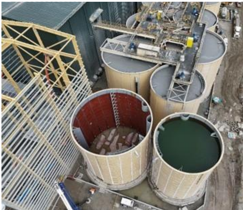
Figure 2 – New leach circuit tanks – July 2026
