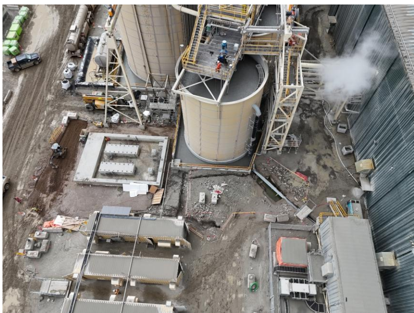
Figure 3 – Shear reactor foundations – July 2026
