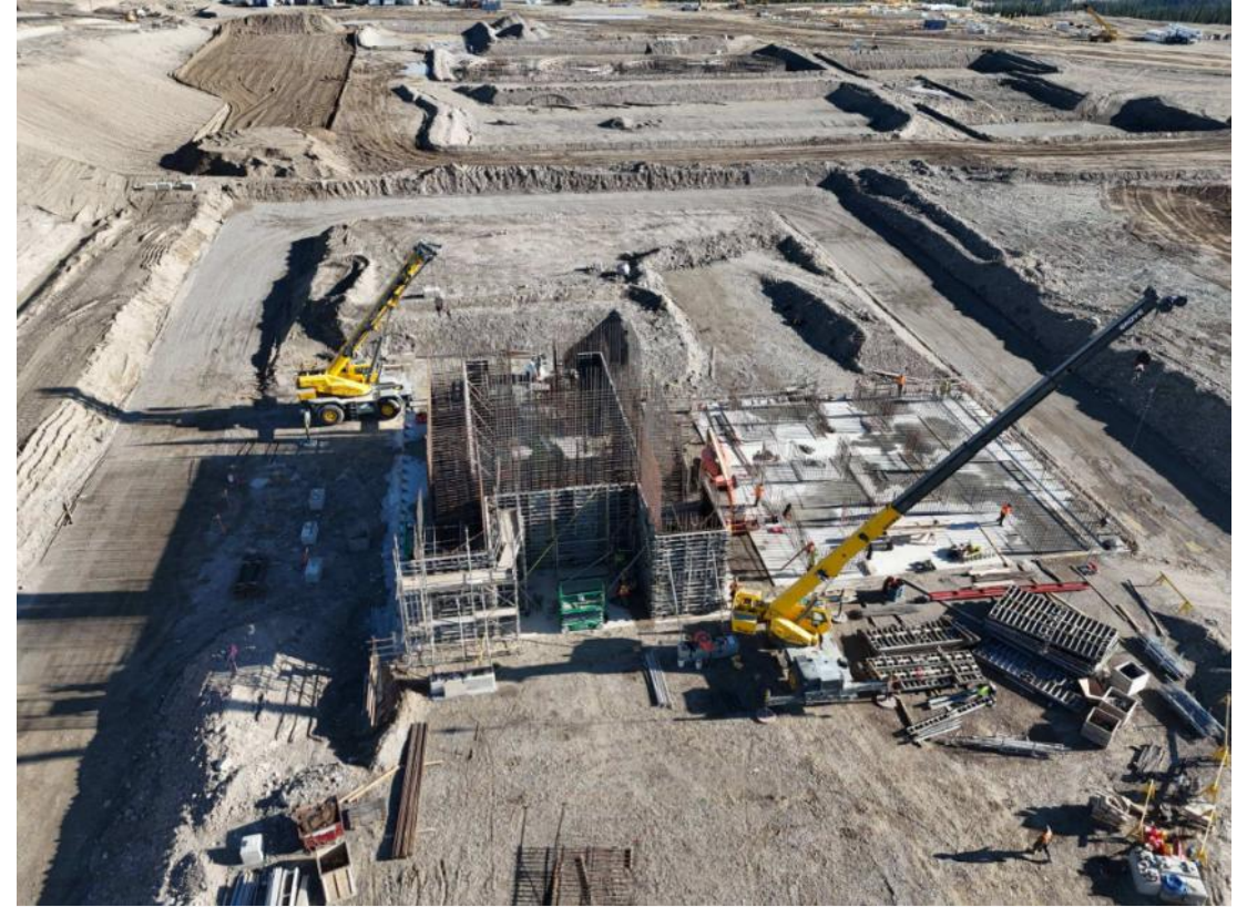
LHS ball mill raft and pedestal (first lift) RHS SAG mill raft. Surrounding area mill building foundation (pre cast) prep – Sept 2026
