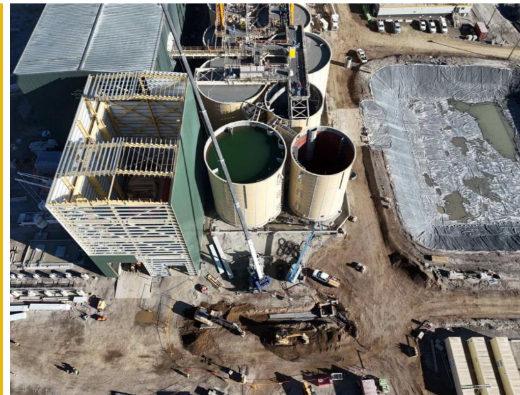
Tower mill building, leach tanks, oxygen plants, switch room and transformers bays completed foundations – Sept 2026
