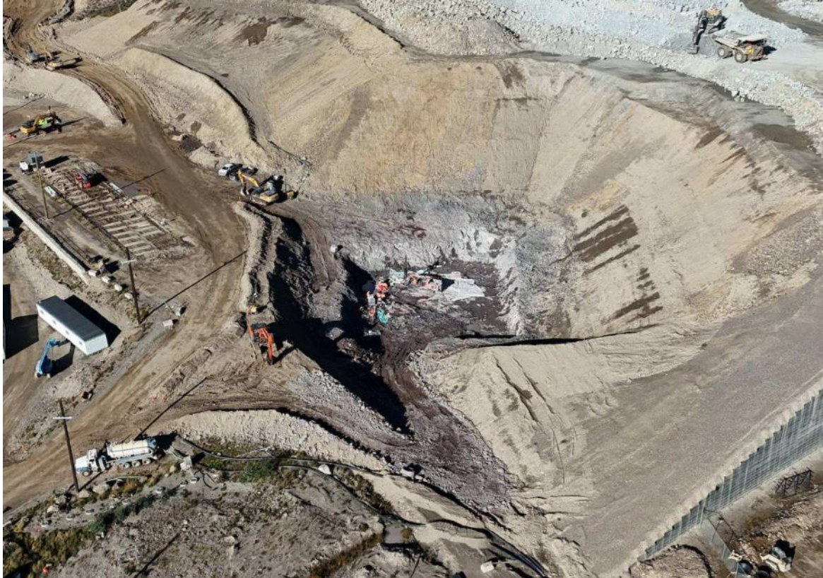
Excavation In bedrock new primary crusher – Sept 2026
