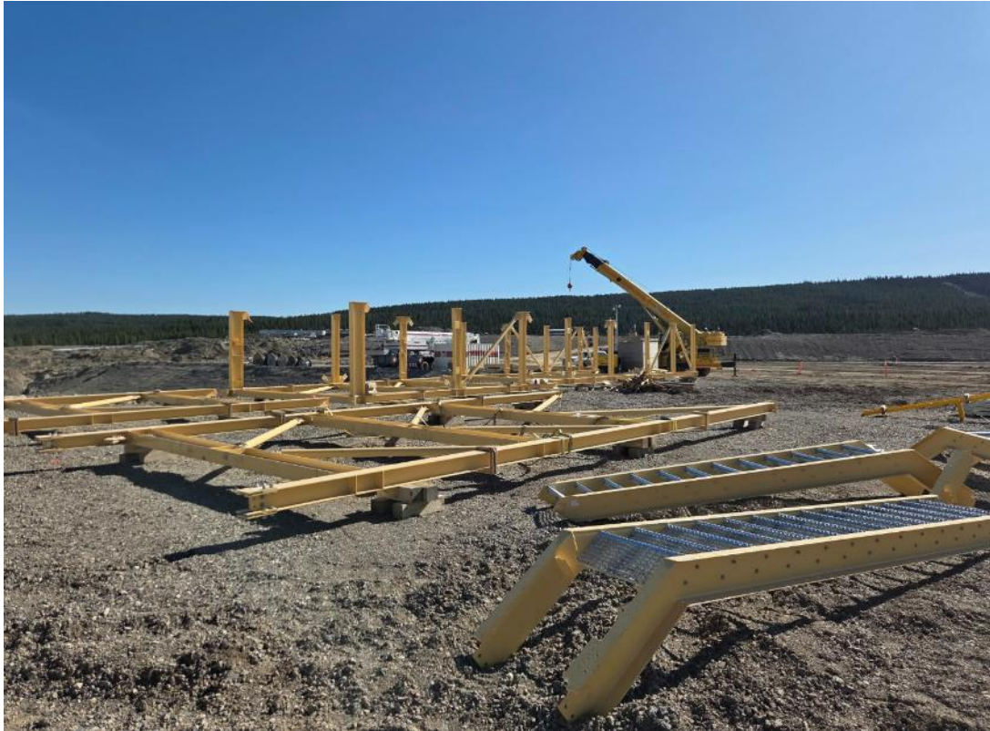
Phase 1A structural steel pre assembly – Sept 2026
