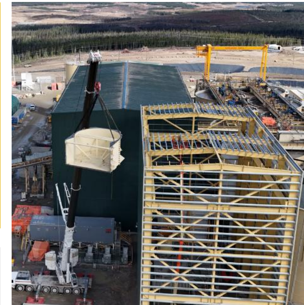
Tower mill body being lifted into place – Sept 4, 2026
