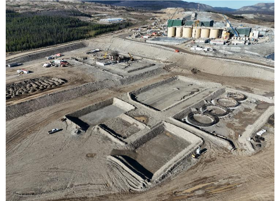
EP2 overview with CIP and leach trains (4 x tank foundation rebar installation) excavations foreground and Phase 1 background
