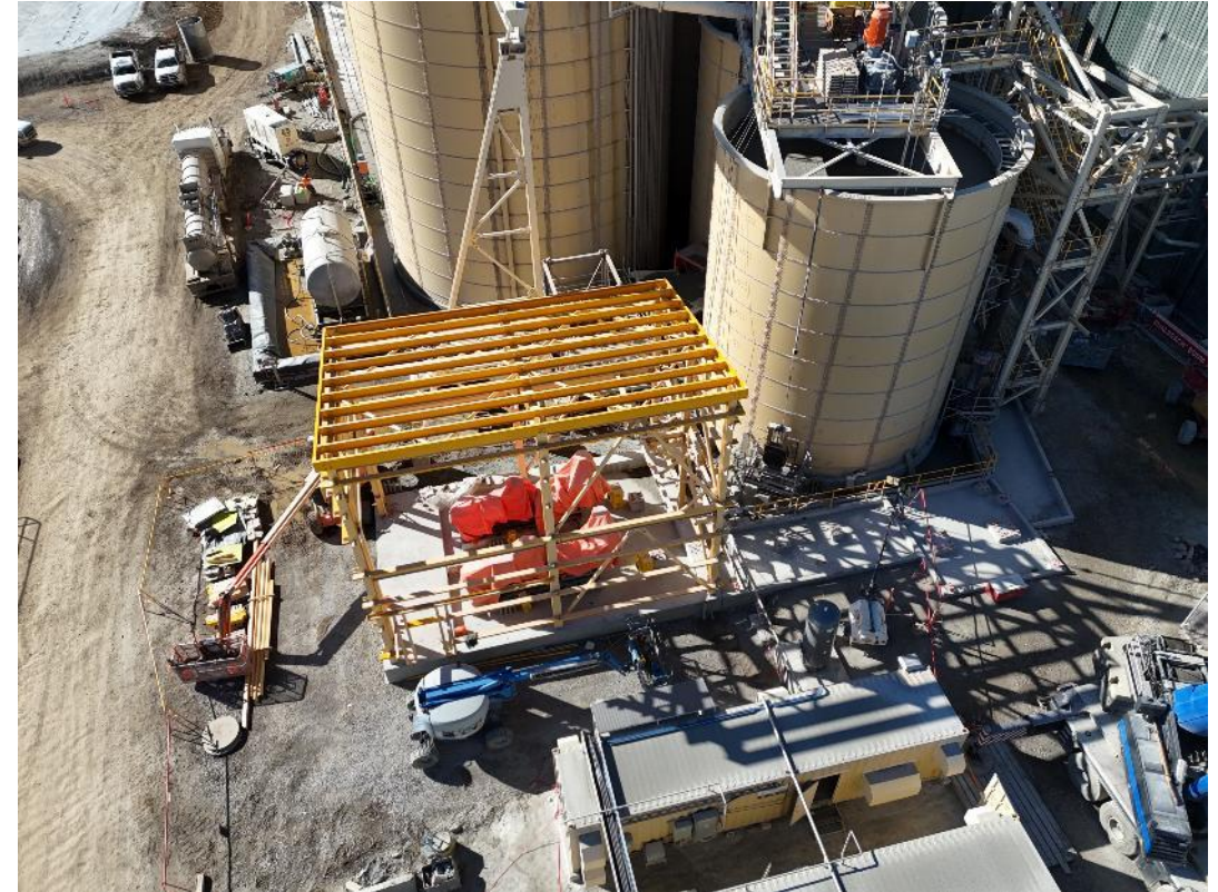
LHS shear reactor pumphouse and RHS structure foundation and containment slab complete – Sept 2026
